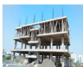
Figure 15. Slab casting 1
